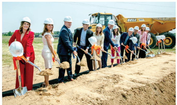
Representatives from Universal Health Services and Trinity Health Grand Rapids broke ground on the new Southridge Behavioral Hospital slated to open in 2025.
